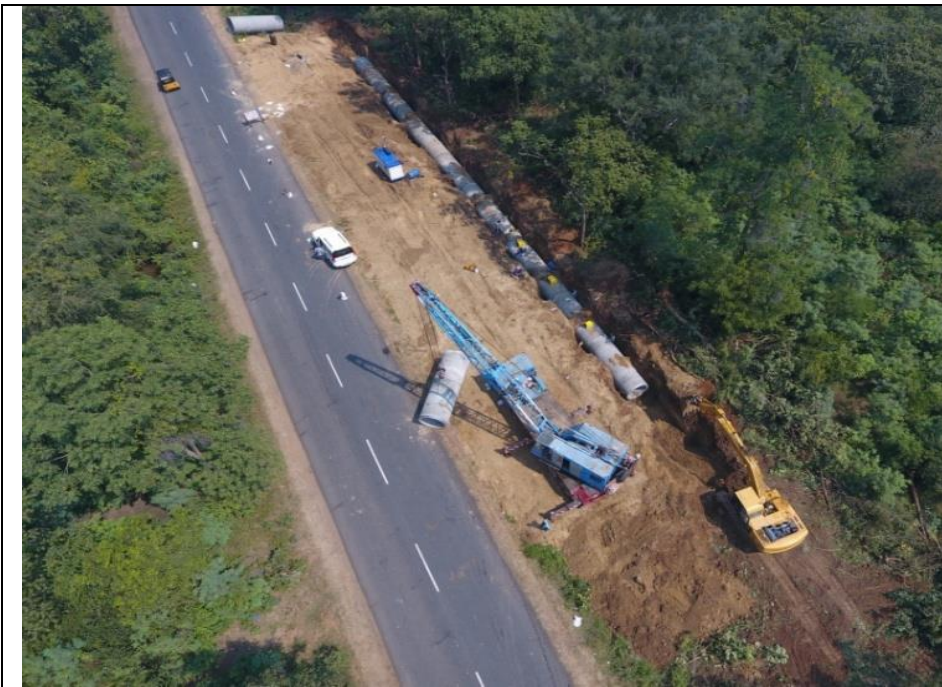
1500 mm dia PCCP Pipeline — Godavari Dummugudem segment
