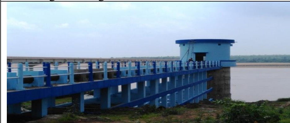
8m dia Intake at Godavari Pusuru (Wazeedumandal) – Pusuru sub segment – KhammamDist
