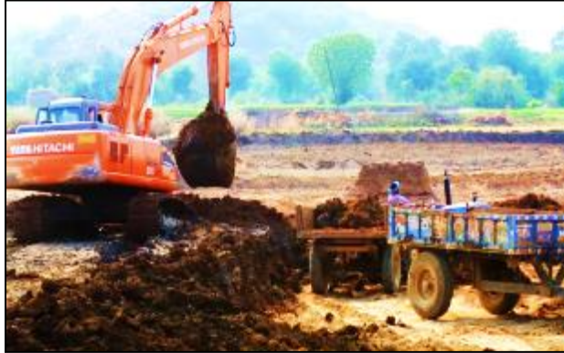
Desilting of the Tank
